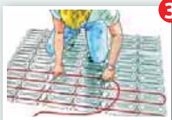
Install heating cable in grooves, pressing gently
